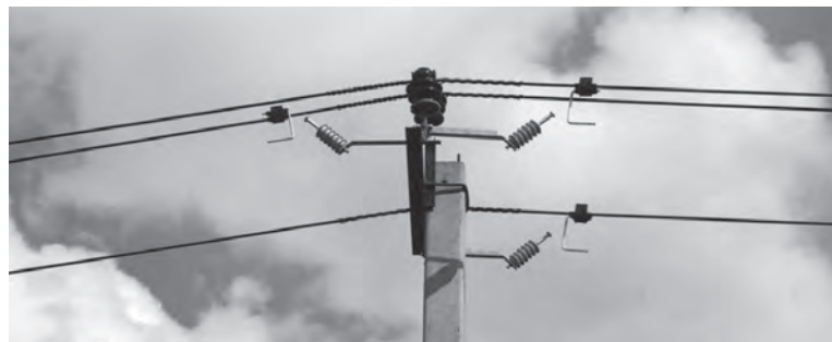
PHOTO. 4. Scheme of installation of APD-EVS-SG on 6-20 kV MV CC for ensuring of possibility of mobile grounding bars connection without installation of additional clamps on wires.
